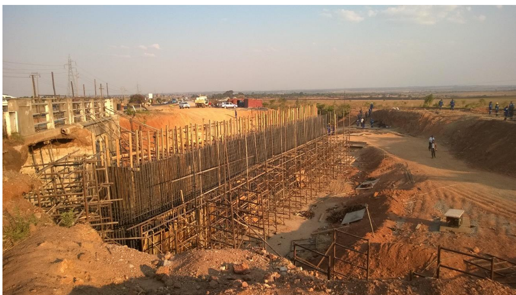
Mabvuku road over rail bridge
