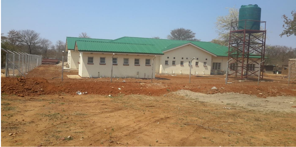
A typical Court House with Legal Aid Offices, Victim Friendly Room, Child Testimony Room & Access ramps for disabled persons, built by the Royal Danish Government
