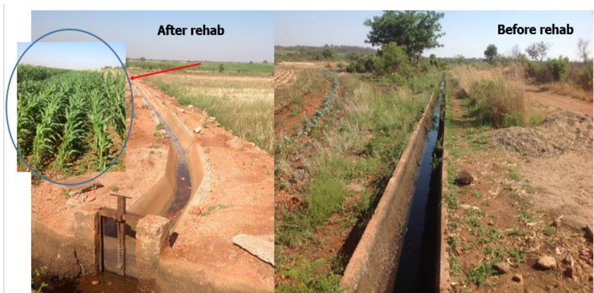
Mhende Irrigation project before and after rehabilitation
