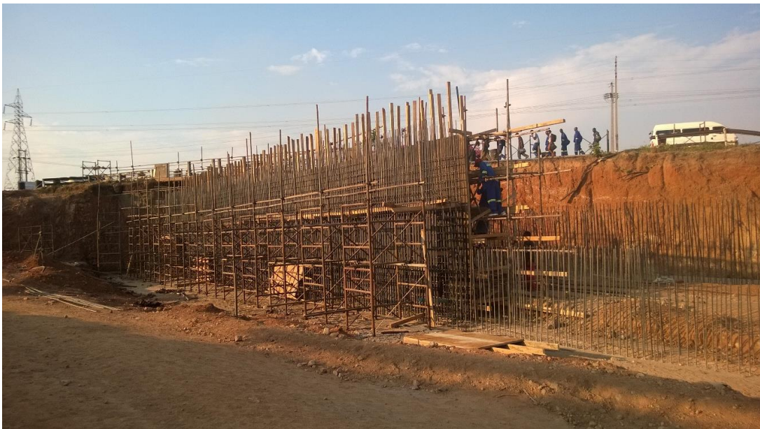
Mabvuku road over rail bridge
