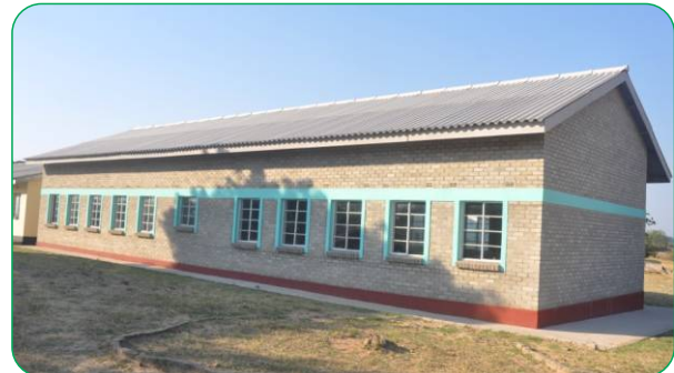
Figure 14: Block constructed by CSOT at Sinami Primary School in Mapanzure
