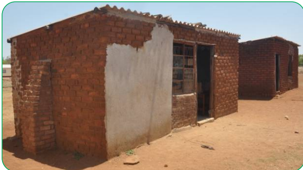
Figure 13: Infrastructure deficit - Mapirimira Primary School in Mapanzure
